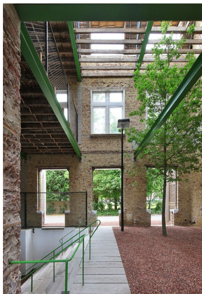
PC CARITAS, Melle, Belgium by architecten de vylder vinck taillieu, © Filip Dujardin
